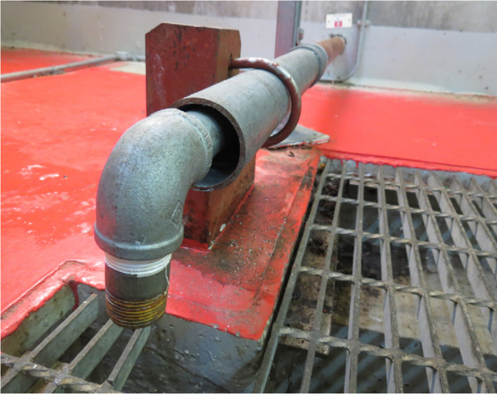
Figure 1.2: Close-up of access.
